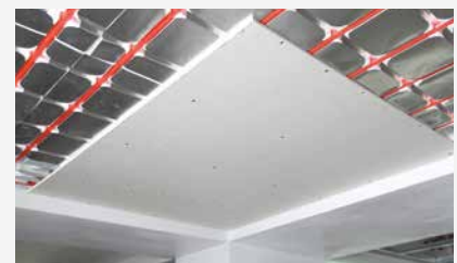
Installation and fitting of plasterboard sheets on the support structure after pressure test performed according to the rules in force
