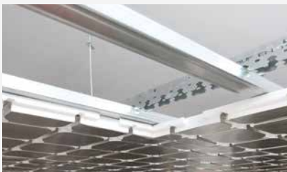
Installation of metal structure with 300 mm pitch
