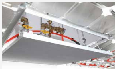
Installation of zone inspection trapdoors where the distribution manifolds are installed
