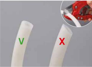
**PIPE CUT.** Square-cut the pipe perpendicularly to its axis taking care not to deform it.
